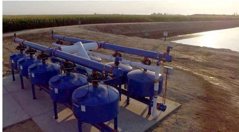
Manure-nutrient water from a storage lagoon goes through an advanced filtration system and is mixed with fresh water before being applied to feed crops via sub-surface drip line.
