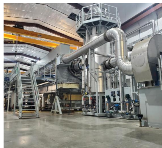
An evaporative system processes liquid manure waste on a dairy. Photo courtesy of Sedron Technologies.
