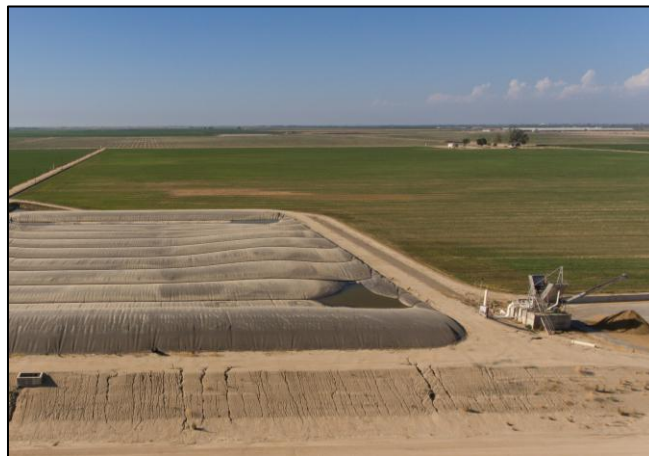
As solid separator (right) removes much of the manure solids before the stream enters covered-lagoon digester.
